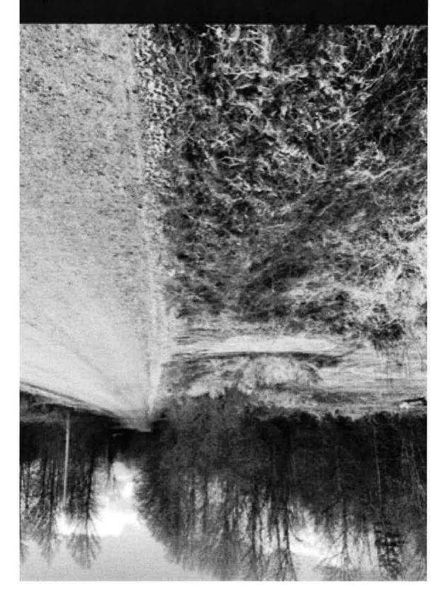
Segment 13605 Morgan Rd. Salisbury before looking uphill. Need to replace driveway culvert, shape and stone line ditch.
